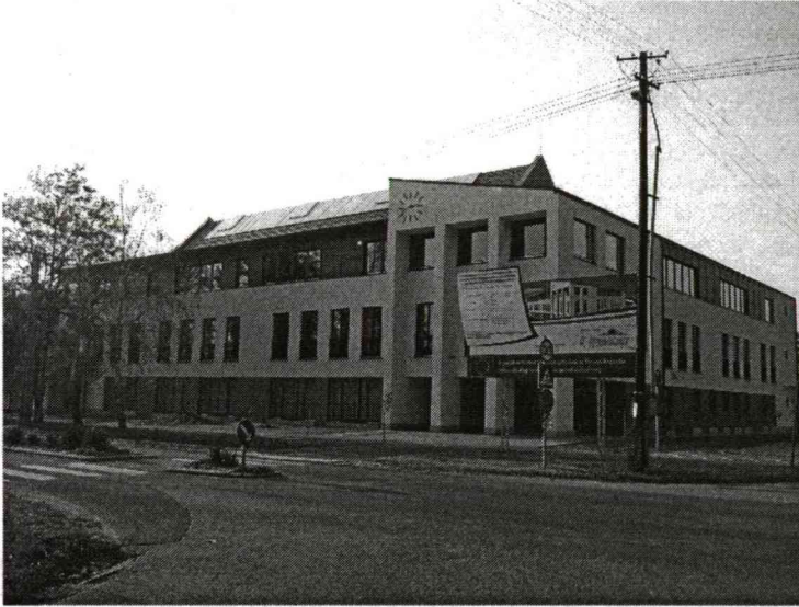
Picture 2. The renovated and amplified school building in the town centre
